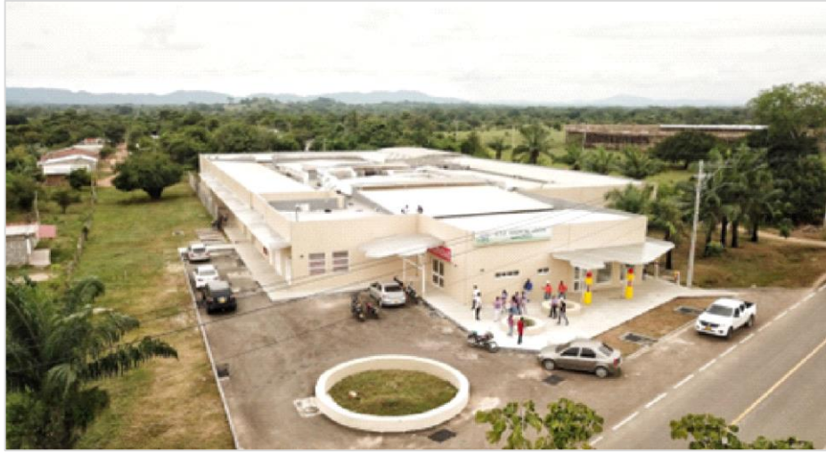
Foto 6. Hospital Local Mahates, Bolívar
